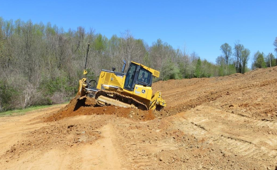
Level-lip spreader during construction
